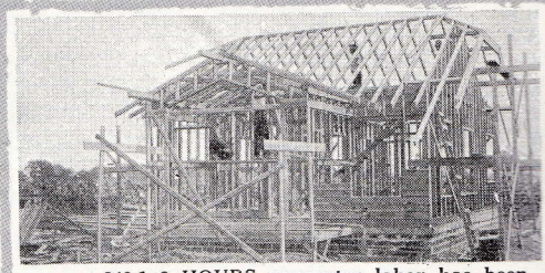
3 243 1-6 HOURS carpenter labor has been spent. Notice how the waste material is starting to pile up. Look at picture No. 3 on opposite page.
